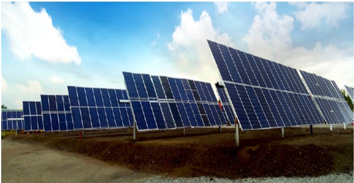
Image 3.2 Typical Single Axis Trackers
