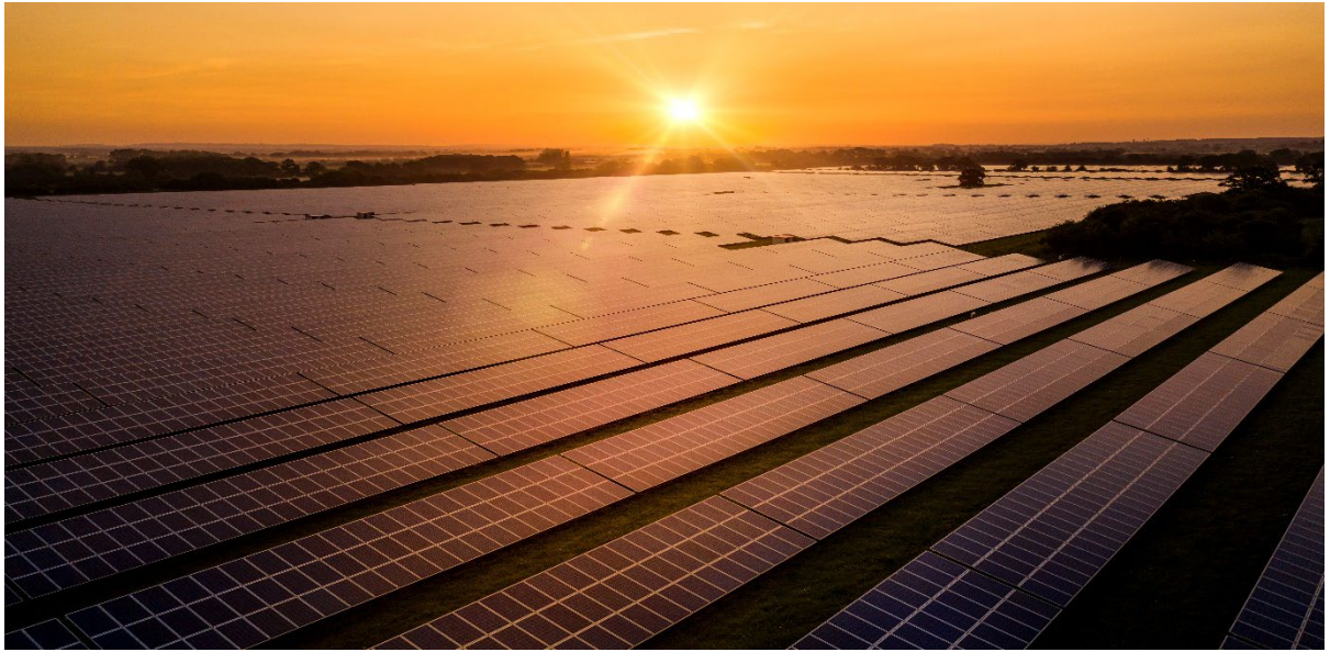
Image 3.1 Typical Fixed South Facing PV Arrays
